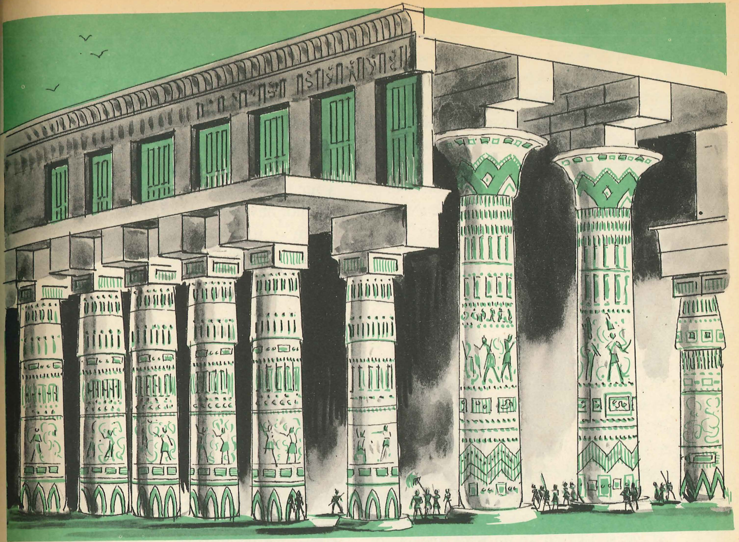
The heavy two-level stone roof of the Great Hypostyle Hall in the temple of Ammon at Karnak was supported by 134 columns arranged in 16 rows. The central rows of columns were 80 feet high.
